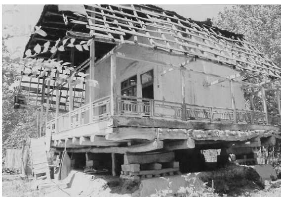
Figure 4. Use of pieces of wood between the ground and the bearing walls of traditional houses in Lahijan, north of Iran. This demonstrates a base isolation technique that was applied long before the introduction of modern base isolation technology.
