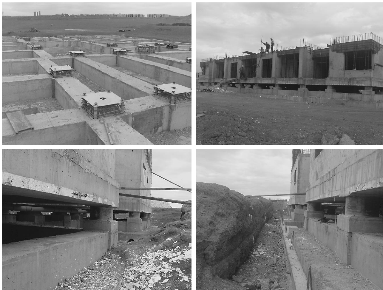
Figure 9. Typical 12 storey base isolated residential buildings under construction in Parand New Town near Tehran.
