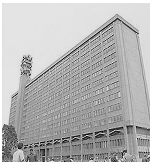
Figure 5. Telecommunication building in the central part of Tehran built in early 1970's. Two Teflon plates with rubber in between are installed between the basement and the ground floor columns of the building.
