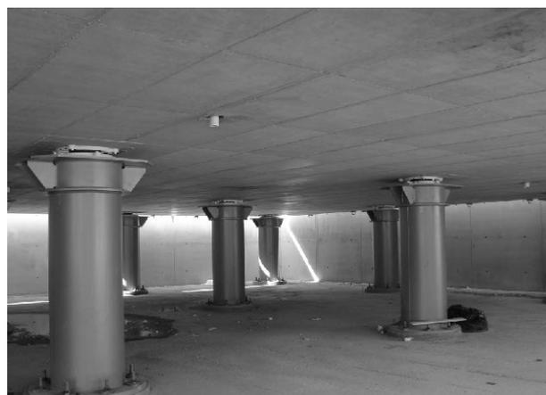
Figure 5. Installed isolation units.
