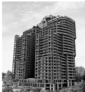
Fig. 7. The 27-storeyed apartment house with seismoisolation system in Kurortny Avenue
