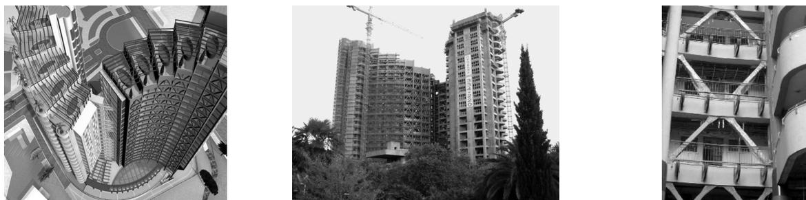
Fig. 10. Apartment housing estate « New Alexandria » with damping system of metal braces
