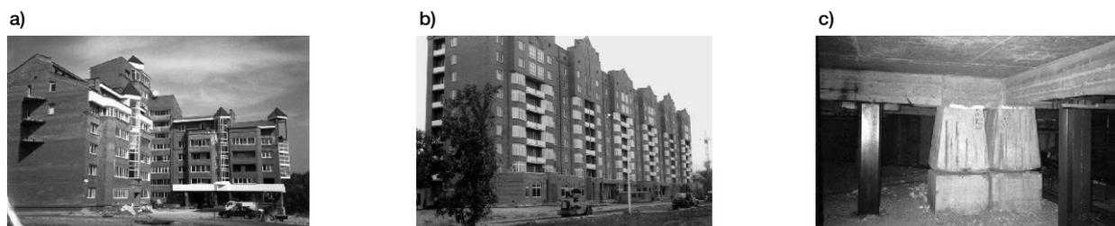
Fig. 2. Seismoisolated buildings: a) in Irkutsk-city; b) in Novokuznetsk-city; c) kinematic rocking supports with hysteretic dampers
