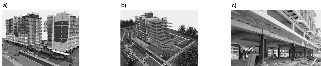
Fig. 3. Application of seismoisolation system in the form of flexible lower story
