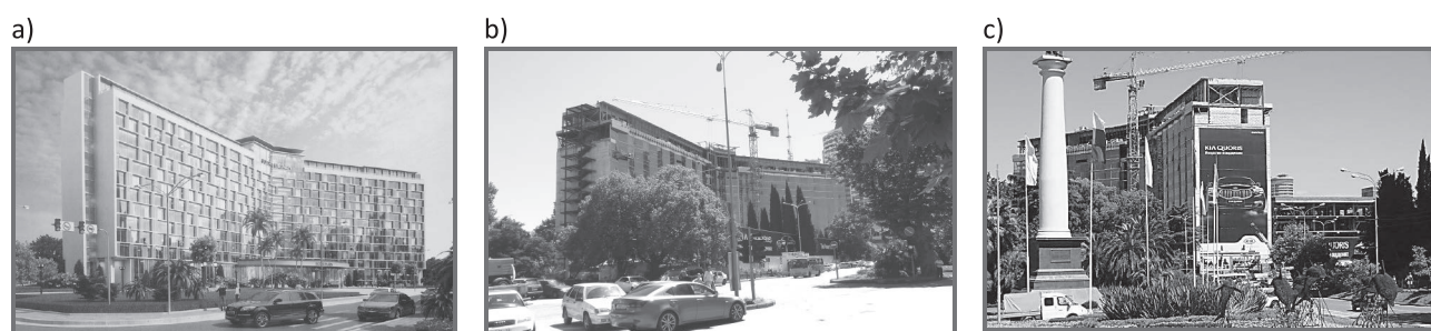
Fig. 5. The Hotel "Moscow" Before and During Reconstruction
