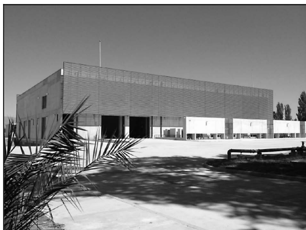
Figure 11. Claro Data Center
