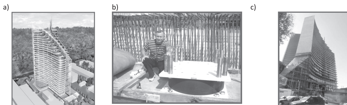
Fig. 8. Hotel building “Hyatt” in Sochi-city a) building facade; b) installation of seismoisolation support; c) the view of the building
