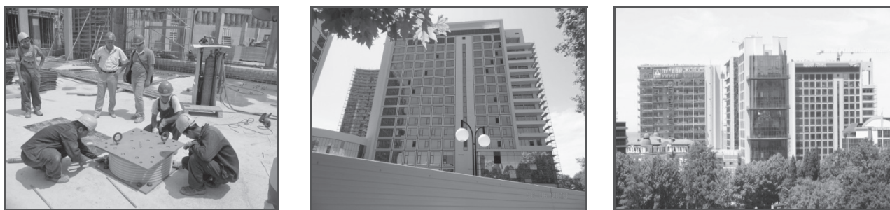
Fig. 10. Russian Olympic university and multipurpose hotel complex a) Installation of RBS on ground floor b) and c) the view of buildings
