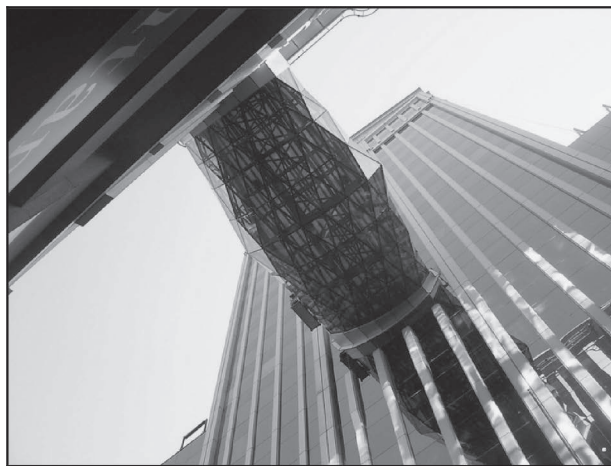
Figure 6. Rubber dampers in pedestrian bridge
