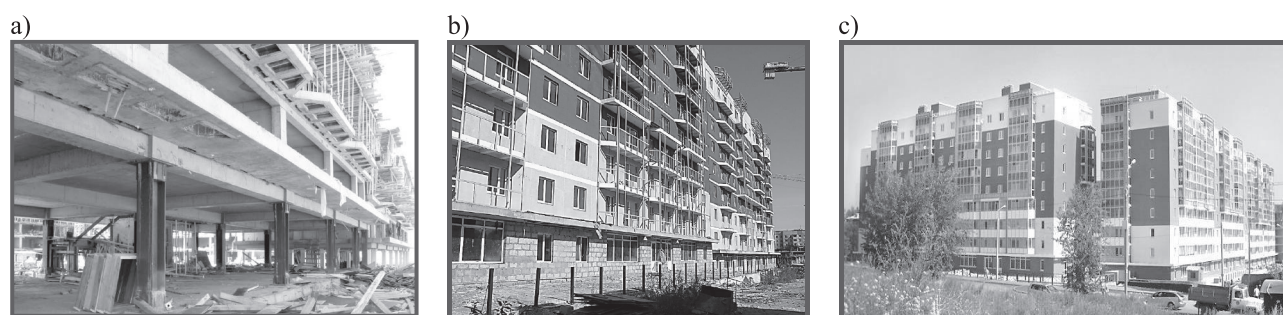
Fig. 3. Application of seismoisolation system in the form of «flexible» lower story a) «flexible» story — metal columns dwelling houses, b) the building under construction, c) the view of the buildings
