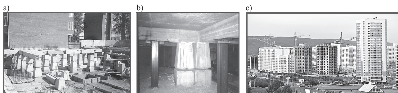
Fig. 2. Seismoisolated buildings a) construction of kinematic rocking supports, b) kinematic supports with metal dampers, c) the view of the buildings
