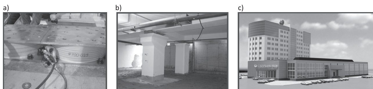
Fig. 12. Bank office building with the system of seismoisolation a) installation of RBS; b) ground floor; c) the building facade
