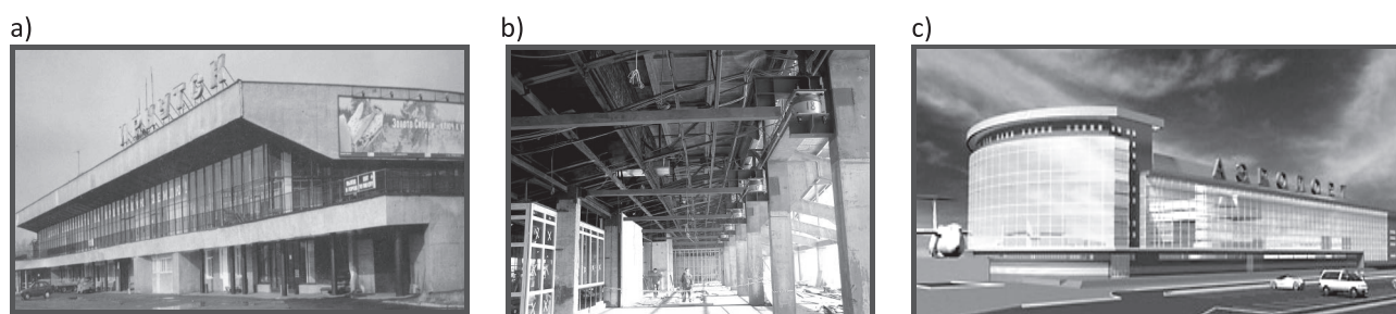
Fig. 15. New solution for seismic protection of the building of Irkutsk Civil Airport a) airport building before strengthening; b) the energy dissipation elements; c) building after reconstruction
