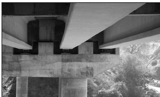
Figure 19. Rio Claro Bridge
