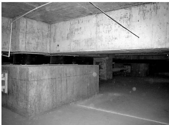
Photo 3. Laminated rubber bearing (Photo; M. Seki)
