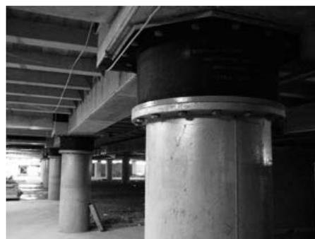
Photo 2. Lead rubber bearings (Photo; D. Whittaker)
