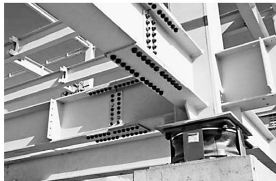
Figure 4- A view of the triple friction pendulum isolator used at the Sabiha Gökçen International Airport (Photo: Prota Inc.)
