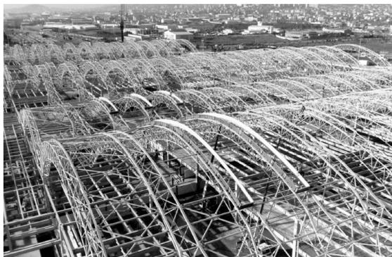
Figure 3- Roof structure of the Sabiha Gökçen International Airport (Photo: Prota Inc.)
