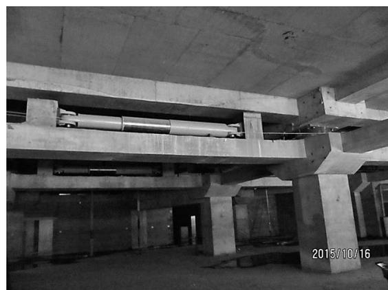
Photo 2. Laminated rubber bearings and oil dampers (Photo; M. Seki)
