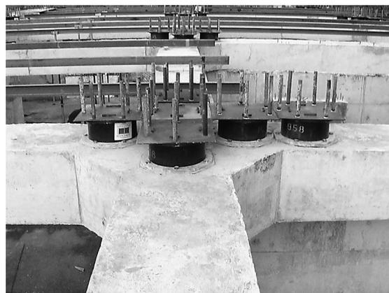
Fig. 4. Example of installation of six rubber bearings under one of the columns of the 18-story base isolated building "Northern Ray" (Photo: M. Melkumyan)
