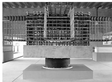
Photo 2 Lead-rubber bearing (Photo; S. J. Wang)
