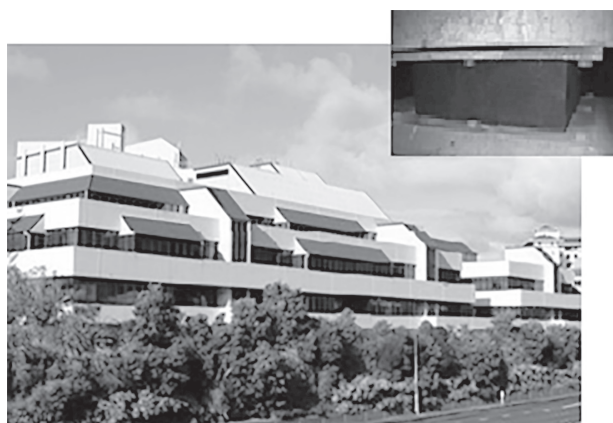
Figure 1. William Clayton building, Wellington
