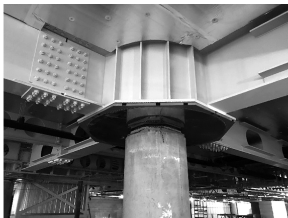
Figure 12. ASB: close view at the isolation level during construction [courtesy of Holmes Consulting LP]
