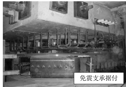
図7 免震化施工手順
